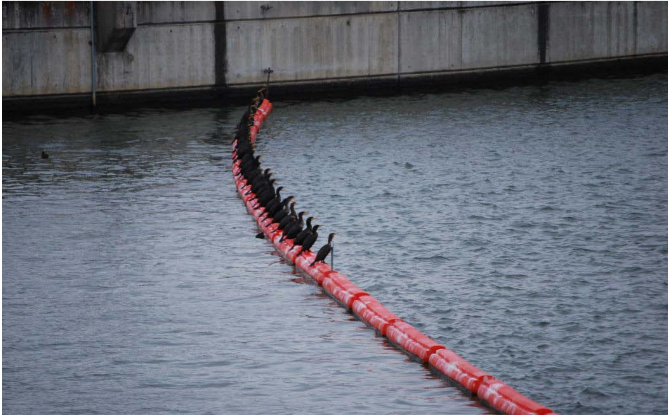
North exit debris boom/cormorant roosting. Primarily a fall/winter behavior. Not as prevalent during spring/summer passage season.
